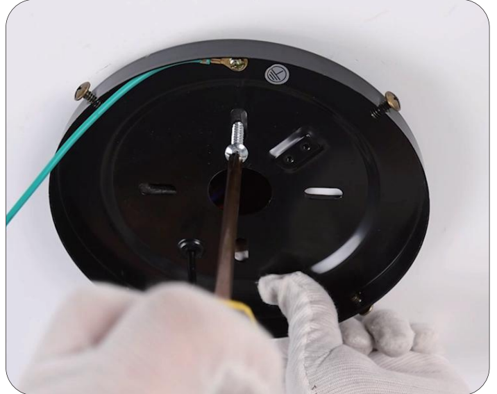
10. Tighten the screws to secure the hanger
