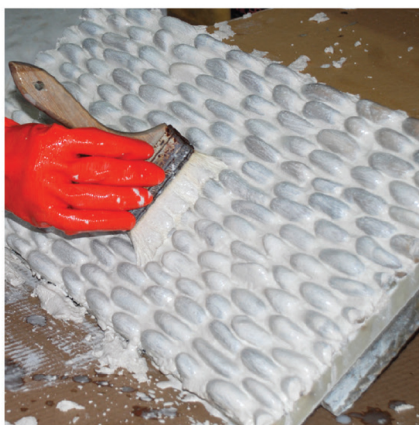
Smooth between pebbles with a paint brush
