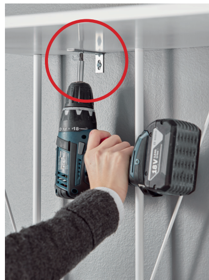
A form of anti-tipping device; angle iron
