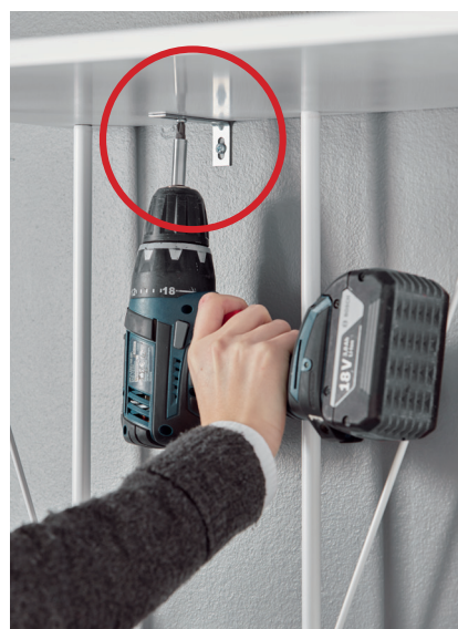
A form of anti-tipping device; angle iron
