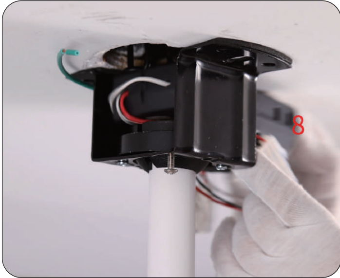
23. Install the Remote Control
