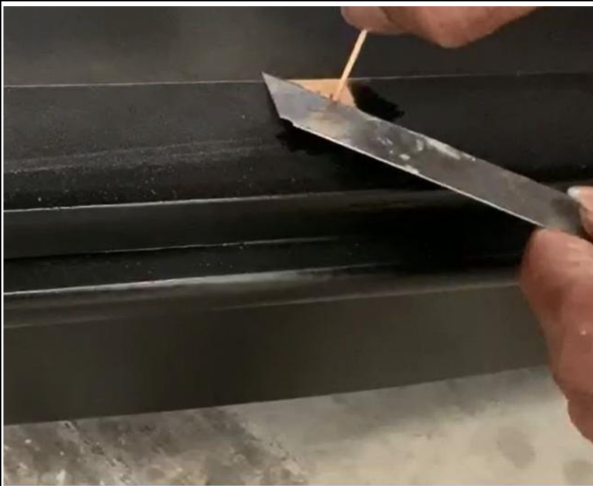
Step 8 Place the blade along the wooden frame and cut off the bamboo toothpick
